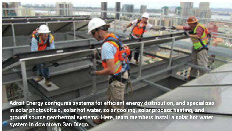
Adroit Energy configures systems for efficient energy distribution, and specializes in solar photovoltaic, solar hot water, solar cooling, solar process heating, and ground source geothermal systems. Here, team members install a solar hot water system in downtown San Diego.
